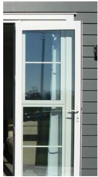
7 White powder coated aluminium window and door frames
