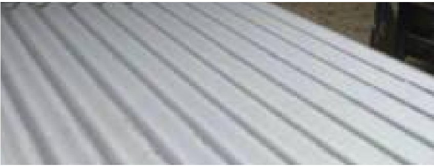
3 Zincalume roofing
